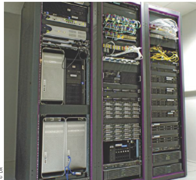
The heart of centralized storage: the 32To Avid ISIS 7000 and the Media Asset Management Avid Interplay.
